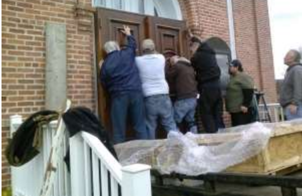
Installing New Doors on Church ↓
