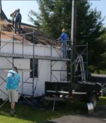
↓ Repair of Garage Roof
